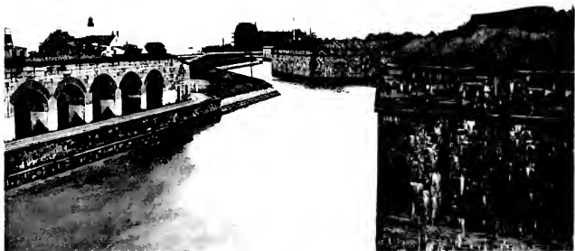
VIEW FROM RAMPARTS, LOOKING WEST.
